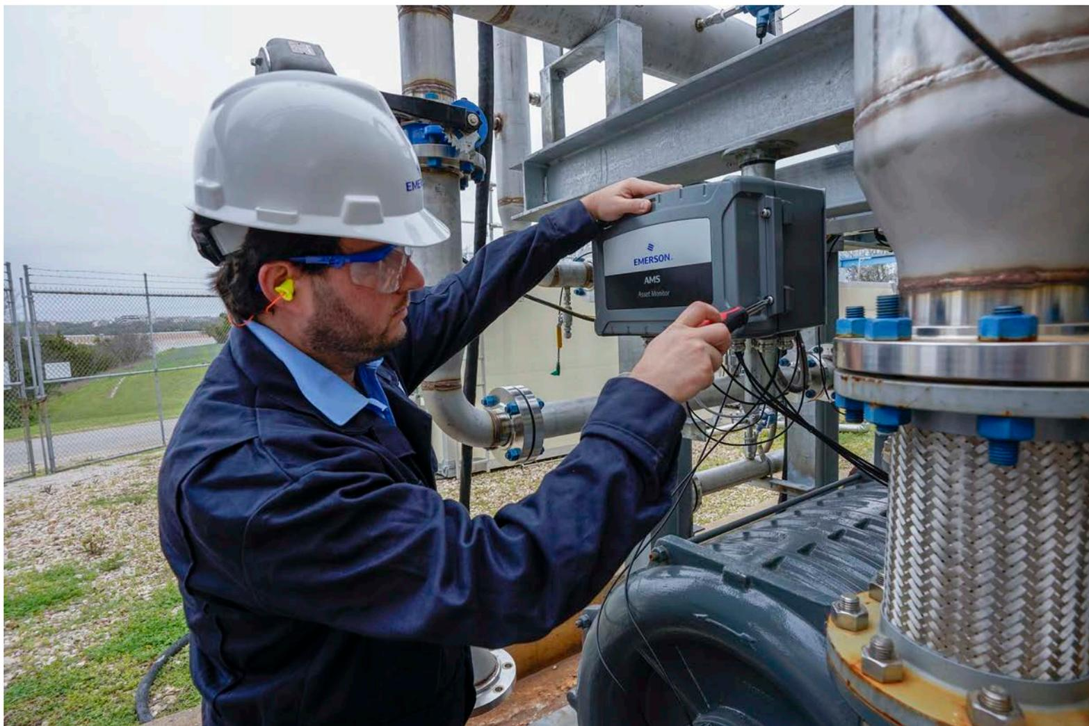
Figure 2: Edge analytics devices like Emerson's AMS Asset Monitor are easy to install right at the asset (Image Courtesy: Emerson)
